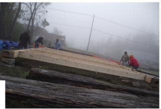
removed from. So at either end of each log a tag had been placed identifying which corner you were working on and the stack order of the log. Thus all of ours bore the label FR (front right). The Bobcat was employed to make sure the logs were on the proper side of the home for stacking and then it was up to us to get them in the right
